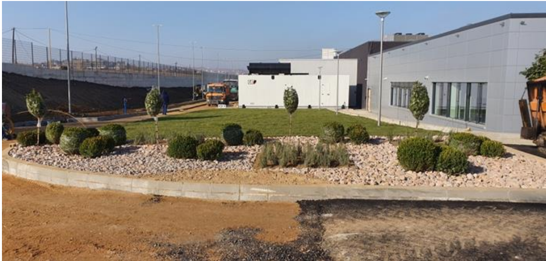
Photo 3. Disaster Recovery Data Center, Phase 1
