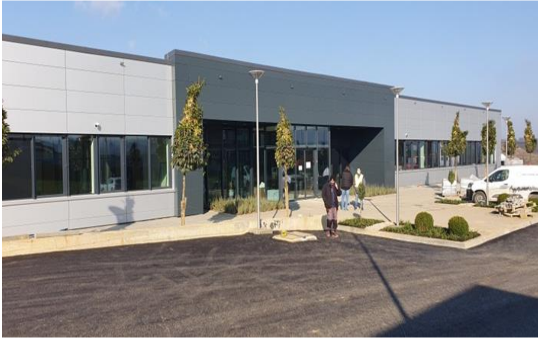
Photo 2. Disaster Recovery Data Center, Phase 1
